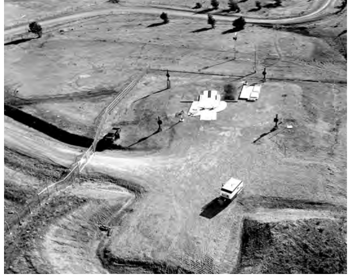
Widely dispersed missile silos were nearly featureless in the open landscape, and most equipment was deep underground. This silo is near Malmstrom Air Force Base, Great Falls, Mont. (Image courtesy of the National Museum of the Air Force)
