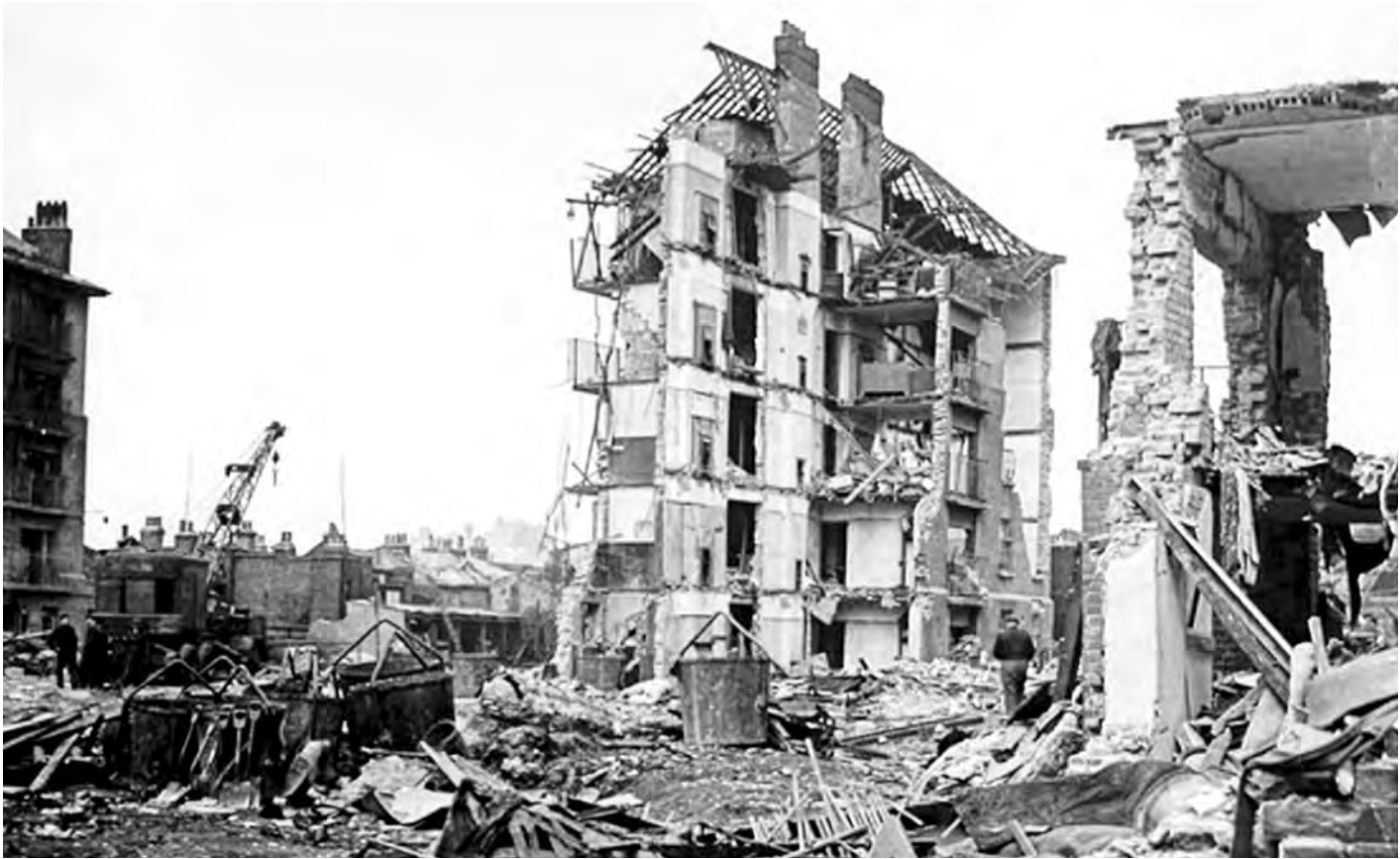
Ruined flats in Limehouse, East London. Hughes Mansions, Vallence Road, following the explosion of the last German V-2 rocket to fall on Greater London, March 27, 1945. Courtesy of the Imperial War Museum. © IWM (HU 88803)
